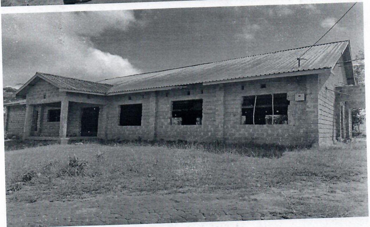
Committee members inspecting the Mutonguni Resource Centre.
