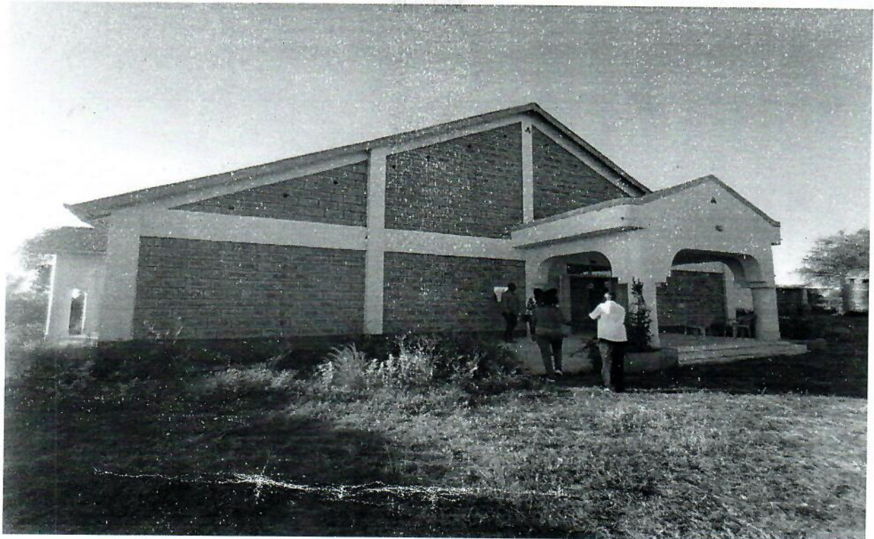
Committee members inspecting the Kyoani Resource Centre.
