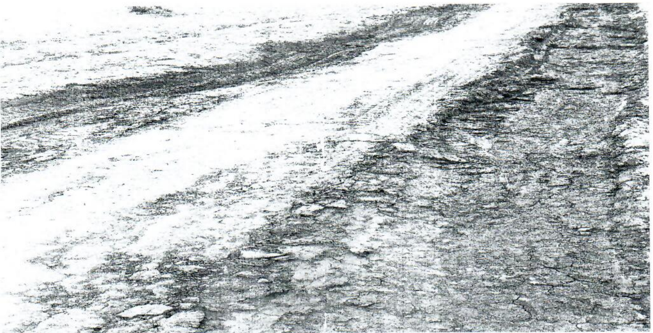
Road washed away by rains
