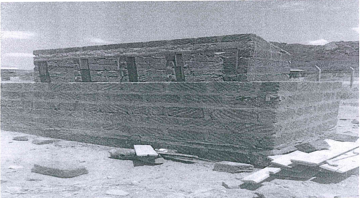
Pit latrine being constructed at Nuu primary Playground.
