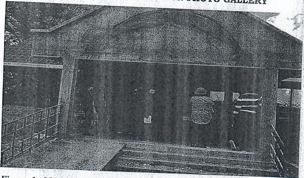
Figure 1. Members inspecting the Lower Eastern Heritage Centre in Tseikuru Ward.
