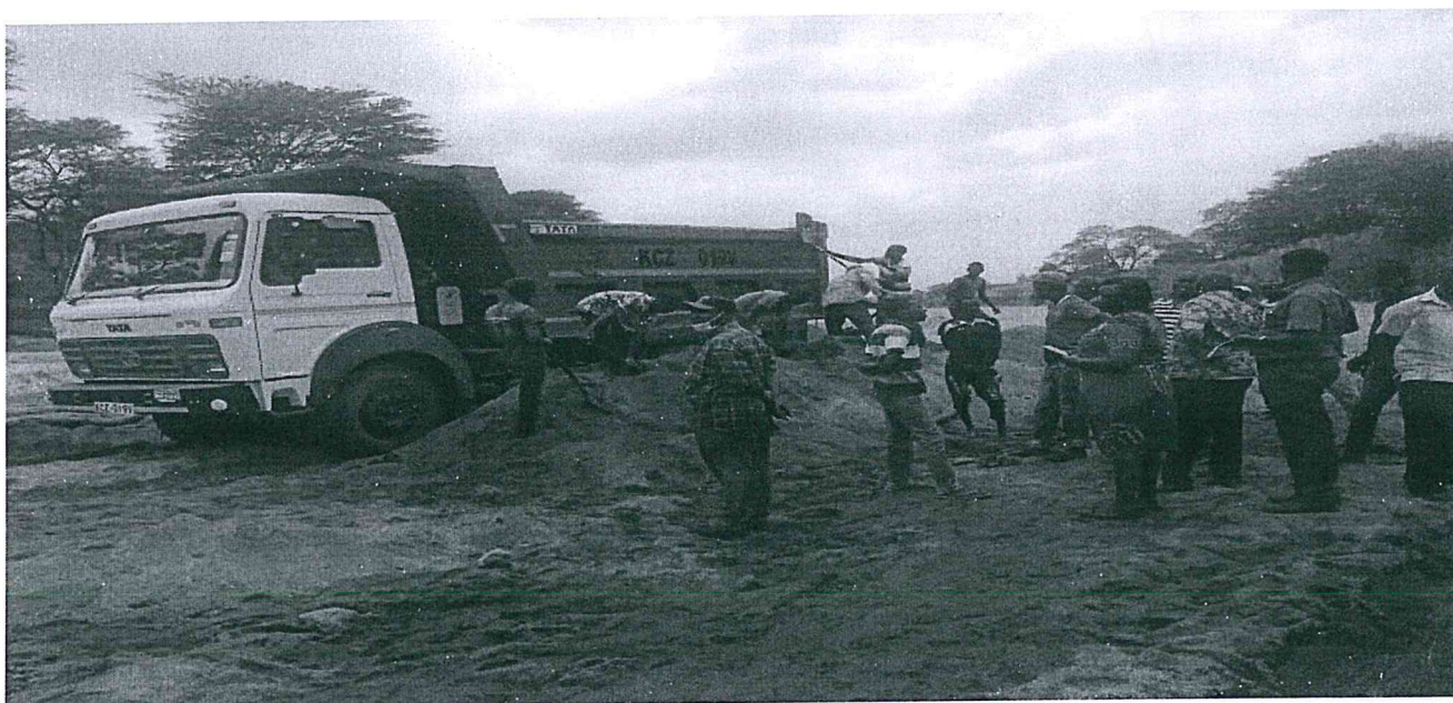
A lorry loading sand at kyusyani site and Members interrogating loaders.
