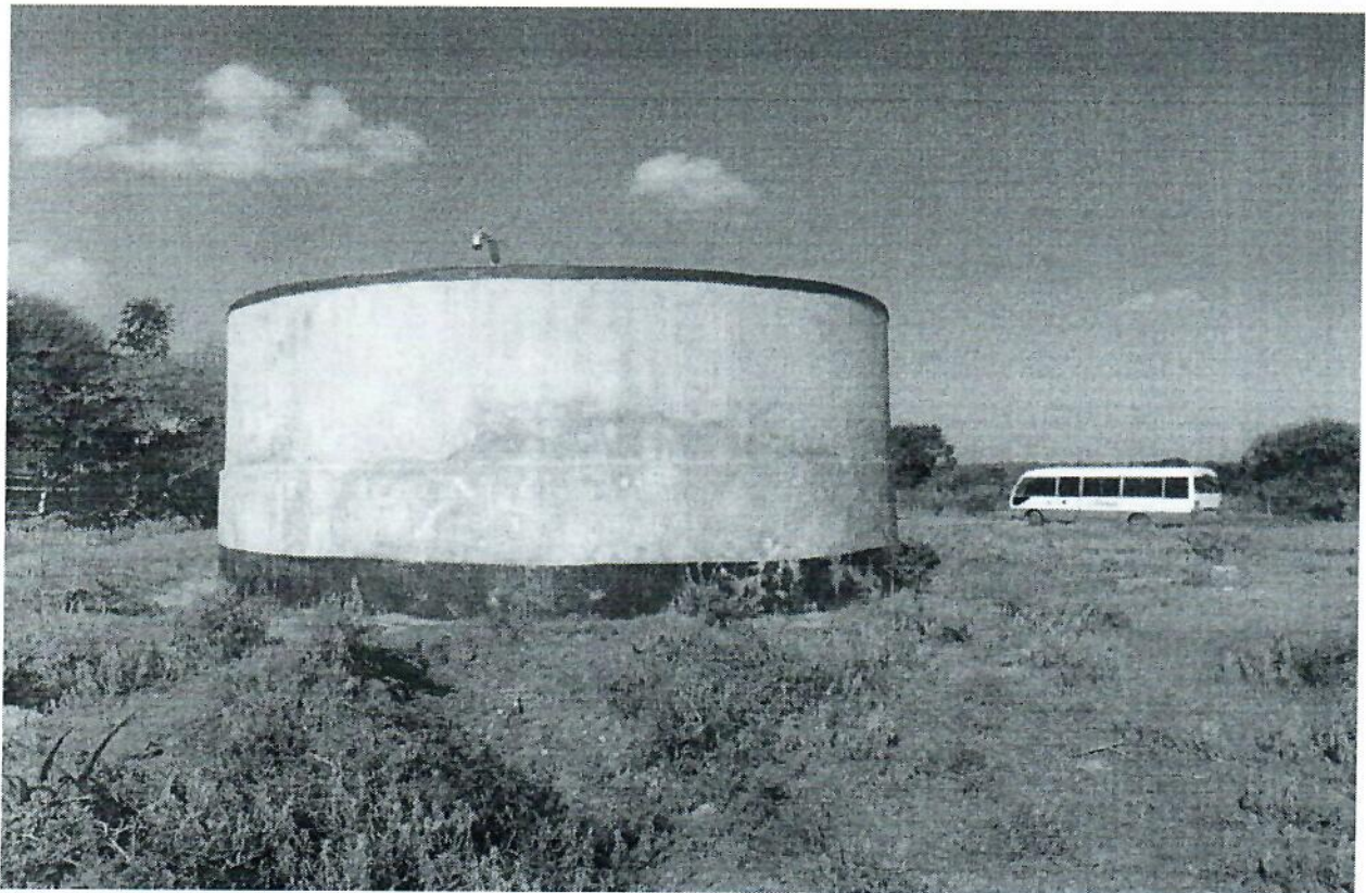
Figure.7.Reservoir Tank and water Kiosk at Kyeng'e Market
