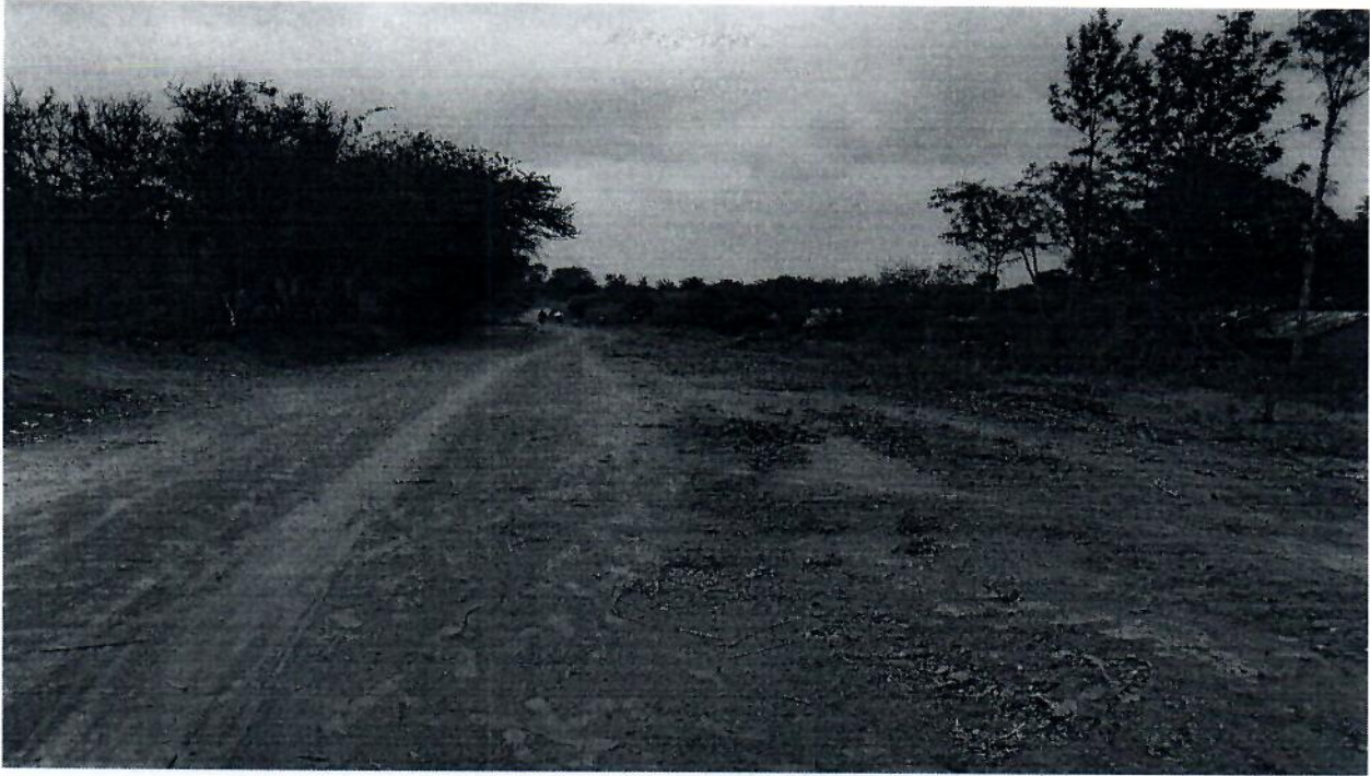
A road section cleared by the Bulldozer at Katheuni Village.
